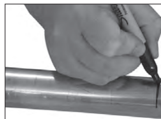
Figure 3 — Marking for Insertion Depth
