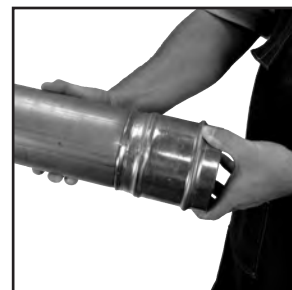
Figure 9: Inspection of final crimp
